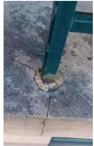
Figure 15: Cracking on Cantilevered Balcony Railing
