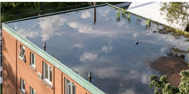
Figure 11: Poorly Drained Roof
