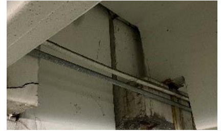
Figure 8: Exposed Rebar
