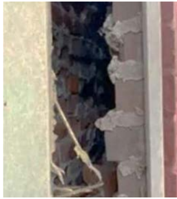
Figure 12: Masonry Wall at Risk of Collapse (CARTA Advisors, LLC)
