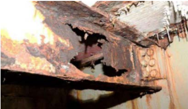
Figure 14: Highly Corroded Steel Beam
