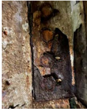
Figure 6: Highly Deteriorated Bolted Connection (CARTA Advisors, LLC)
