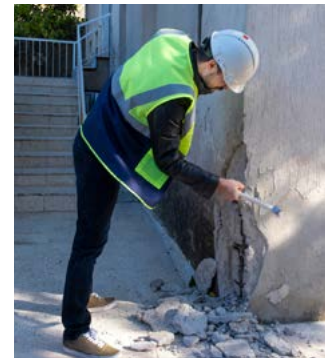
Figure 2: Exposed Rebar
